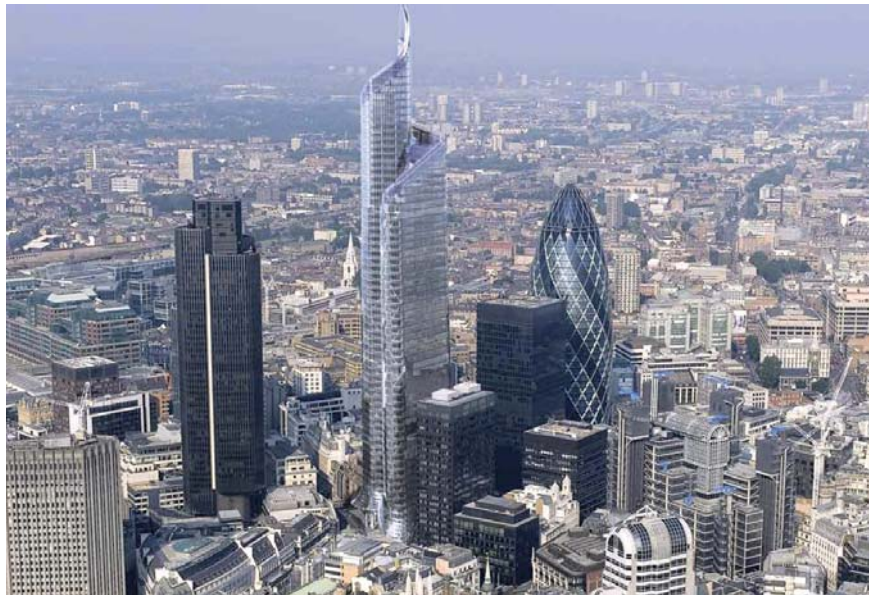
Mace Group is project managing the delivery of The Pinnacle, a 60 floor, 300m high commercial office tower in the City of London (artist's impression)
