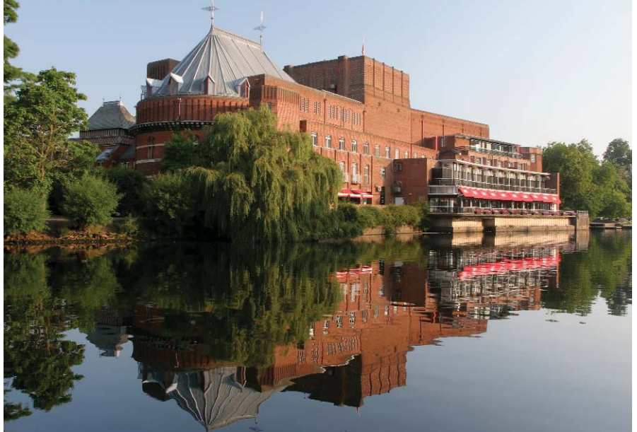
Mace Group is construction manager on the Royal Shakespeare Company's theatre transformation project which involves partial demolition and rebuild of the Grade II* listed theatre to provide a thrust stage auditorium
